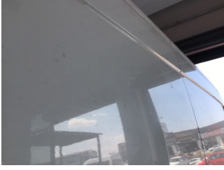
Çamurluk, sol, Çamurluk, sol > Ezik
